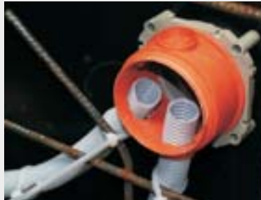
Flexible pipes installed into KBT body.
