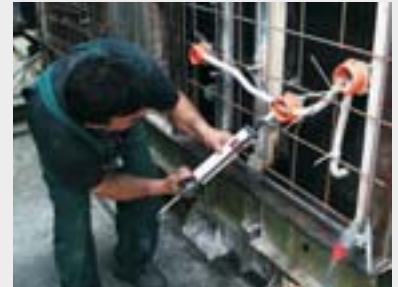
Sealing the penetrations (mastic).
