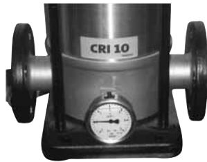
Fig. 59 CR pump with pressure gauge
